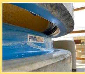
FULLY LINED MANHOLE INCLUDING JOINT LINING
