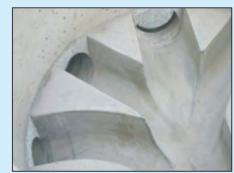
Frequently the question is asked whether and how additional connections can be implemented to a manhole with PREDL®-base-liner. In principle can be attached additional connections at each manhole with PREDL®-base-liner. Because manholes with PREDL®-base-liner have a very high concret-quality, you only need to drill a hole of the size of the incoming pipe.
